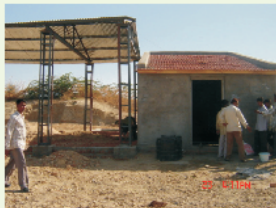
A gasifier work shed and biomass storage room in Vavdi village
