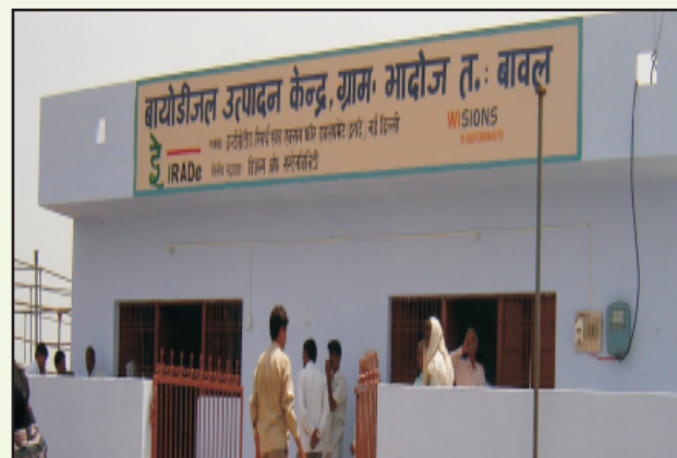
Building of Biodiesel Extraction Unit, Bhadoj, Bawal
