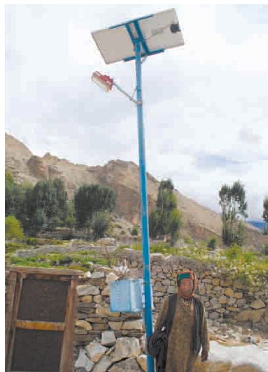
Solar Photovoltaic System in Himachal Pradesh
